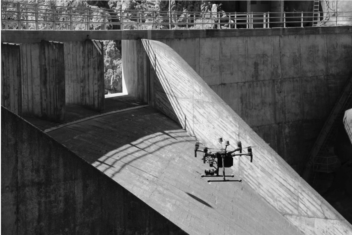
Figure 4. UAV for close range photogrammetry of dam surface.
